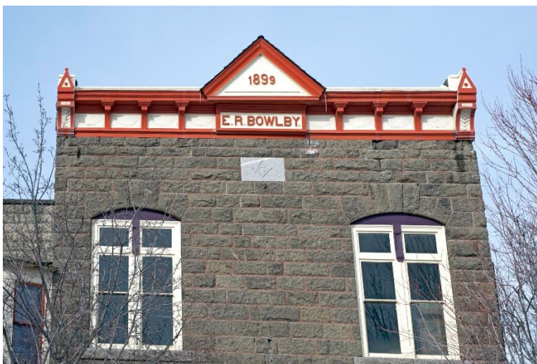
Bowlby Stone on the Bowlby Building in Enterprise was created in the Wapshilla Ridge flow. Photo by Ellen Morris Bishop.
