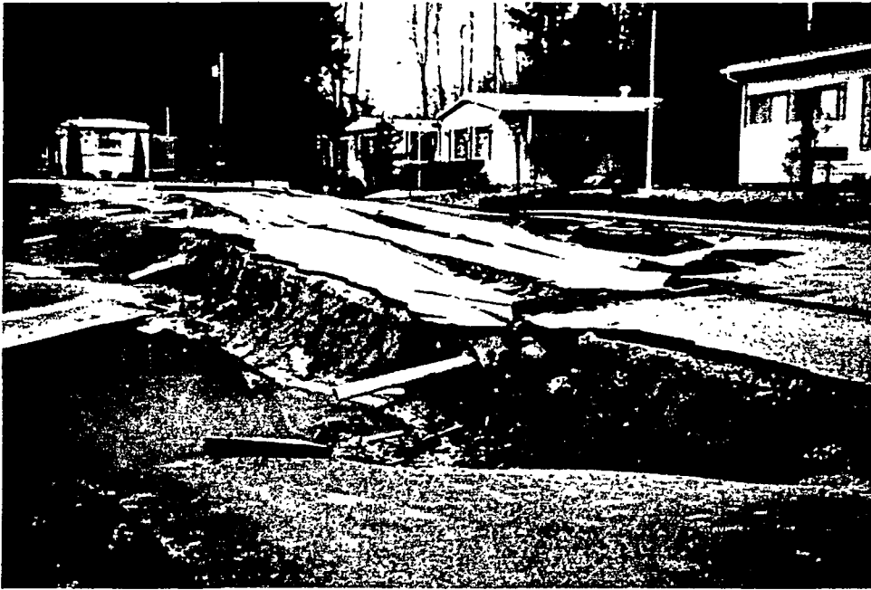
Lateral Spreading at Sunset Lake Mobile Home Park
