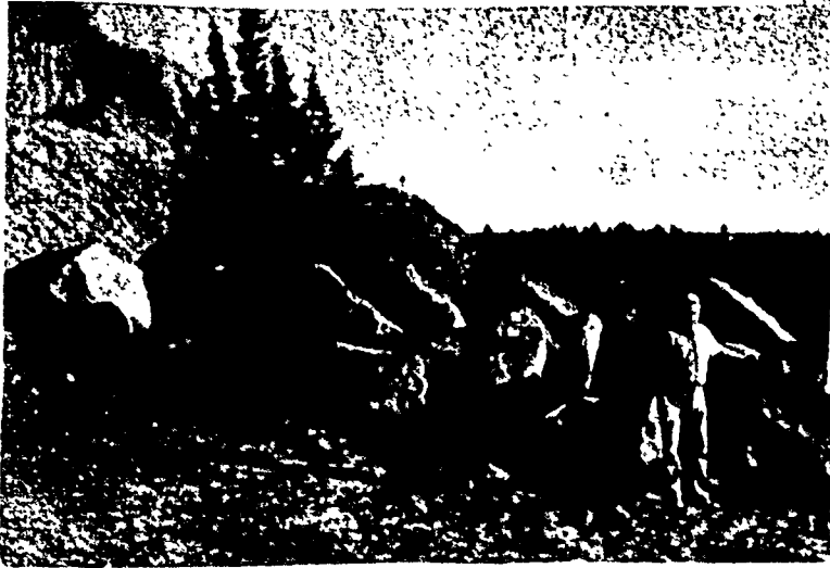
Figure 6. View of the landslide that forced a change in excavation plans. The entire slope of topsoil below the road began to creep as indicated by the visible cracks (arrows).
