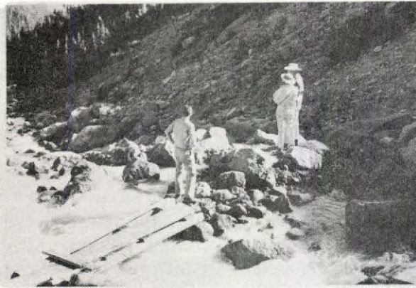
Eliot Creek Bridge
