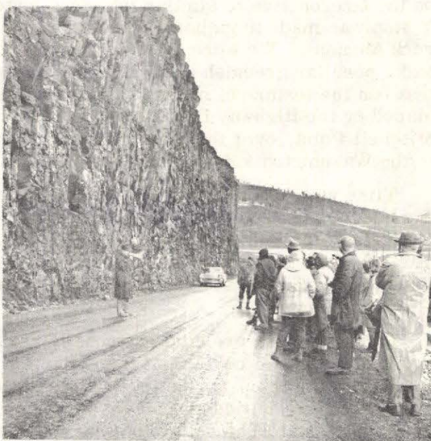
Paul Howell and Lloyd Wilcox point out fault zones, breccia and slickensides, 71.6 miles
