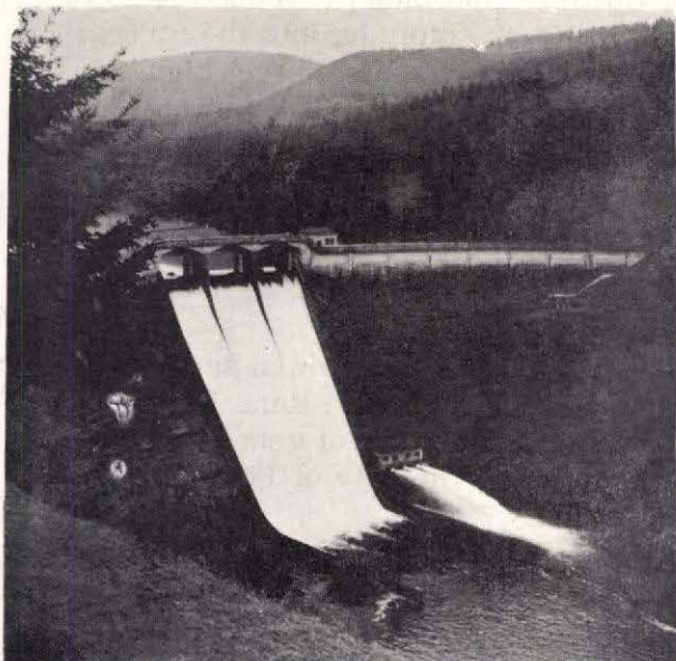
No. 1 Dam of the Bull Run Water System built in 1929 at Bear Creek holds 9 of its 10 billion gallon capacity in Lake Ben Morrow
